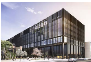
Manchester Engineering Campus Development, UK
