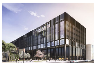
Manchester Engineering Campus Development, UK Size: 81,000 m 2 Year: 2014 - 2020
