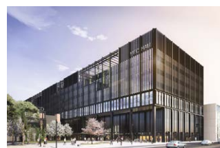
Manchester Engineering Campus Development, UK Size: 81,000 m 2 Year: 2014 - 2021
