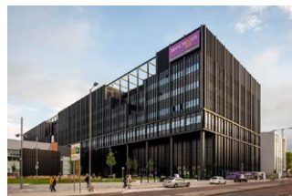
Manchester Engineering Campus Development, UK
