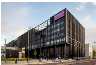
Manchester Engineering Campus Development, UK
