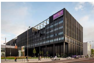
Manchester Engineering Campus Development, UK
