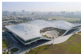
National Kaohsiung Centre for the Arts, Taiwan
