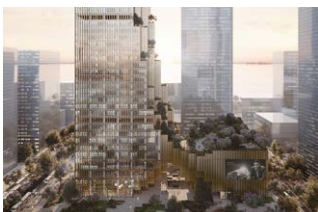
Hengli International Building, Shenzhen, China
